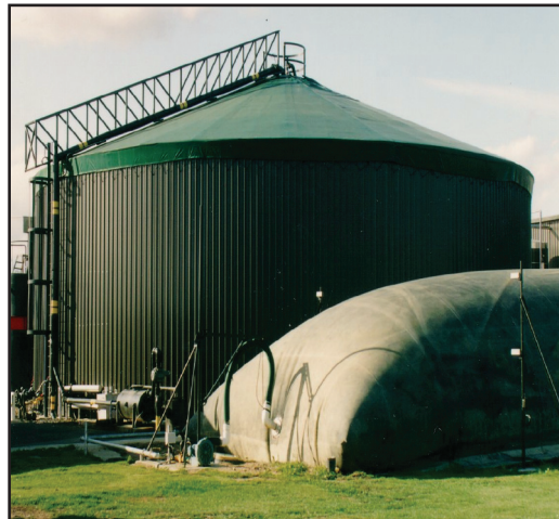
Figure 1 Methane capture at a Brazilian landfill
