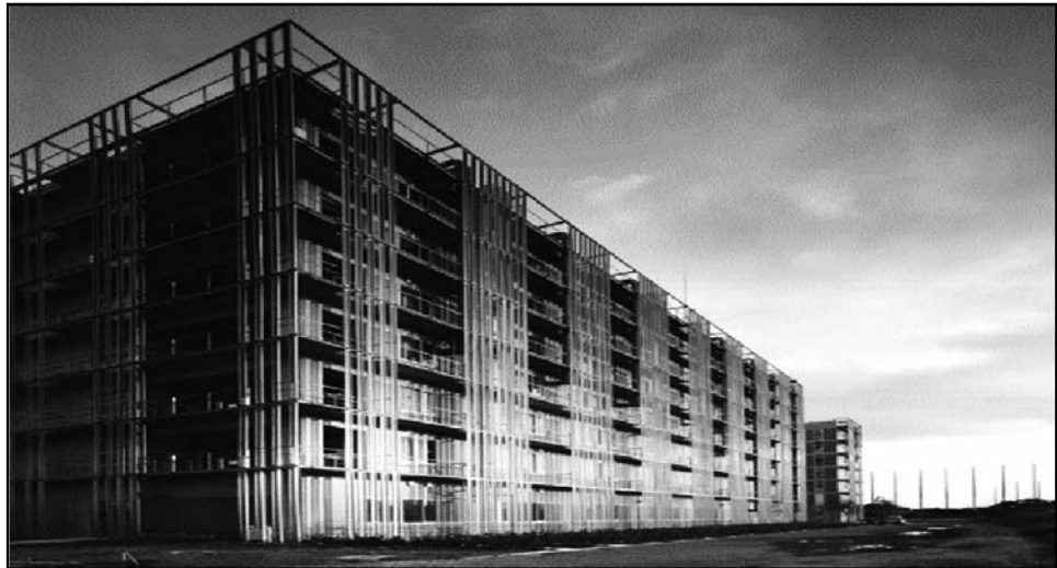
Figure 4 Building envelope showing the louver design for energy savings – Kashiwa Campus, University of Tokyo
